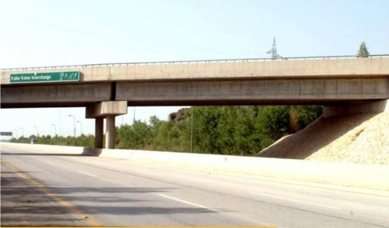
POST TENSIONED BRIDGE – MOTOR WAY PAKISTAN
