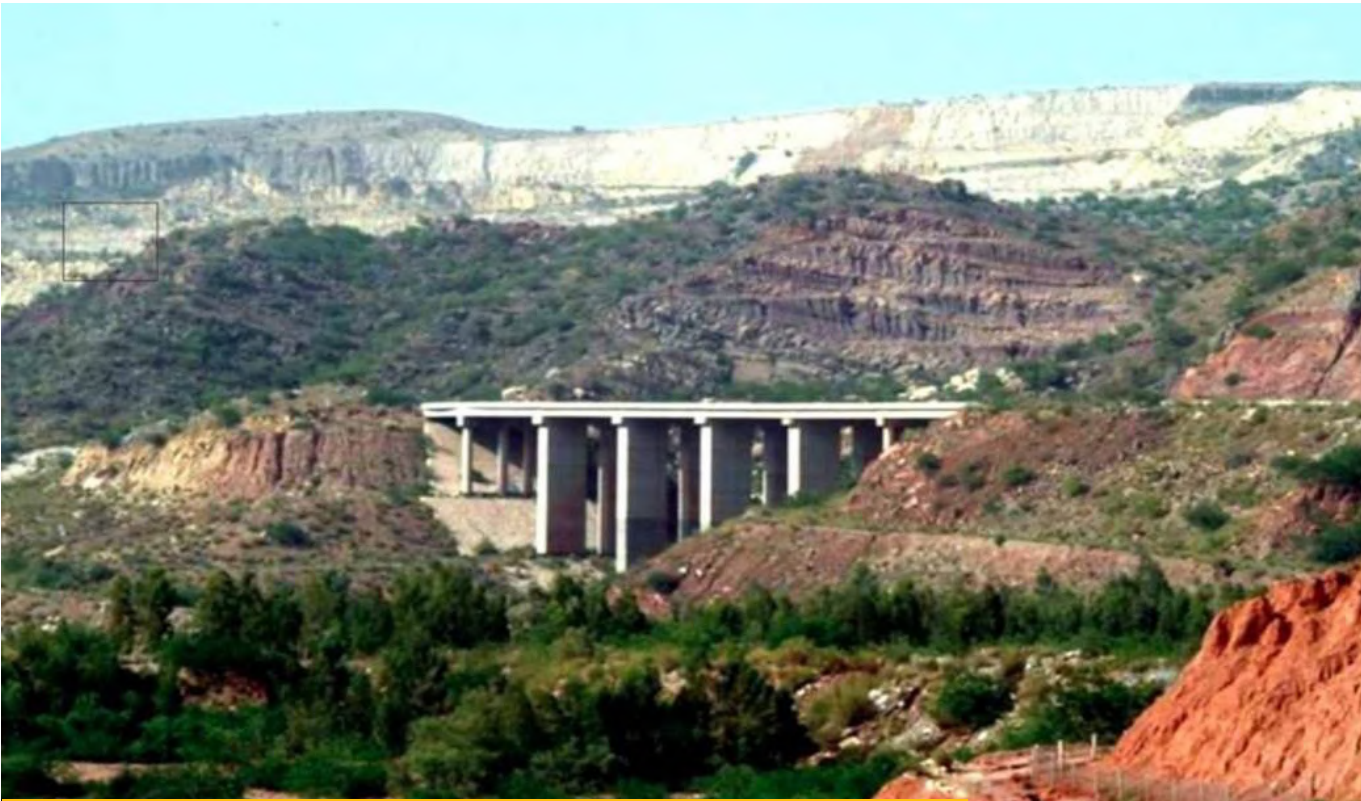
POST TENSIONED BRIDGE – MOTOR WAY PAKISTAN
