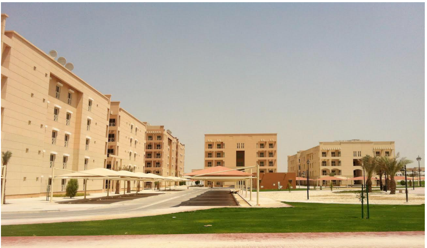
CONSTRUCTION OF TYPE B HOUSES IN BARWA CITY – PHASE 1
