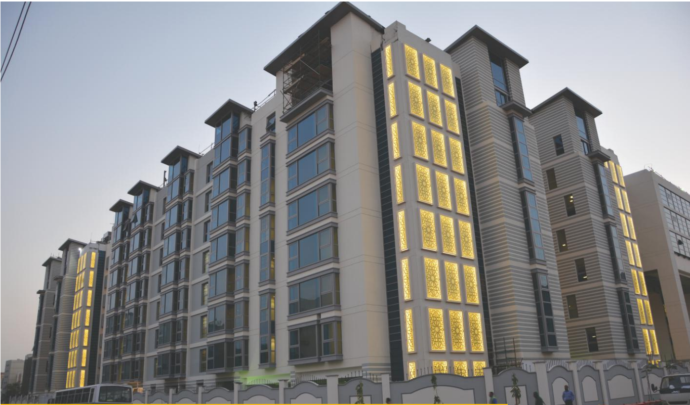
QATAR AIRWAYS – CREW ACCOMMODATION PROJECT
