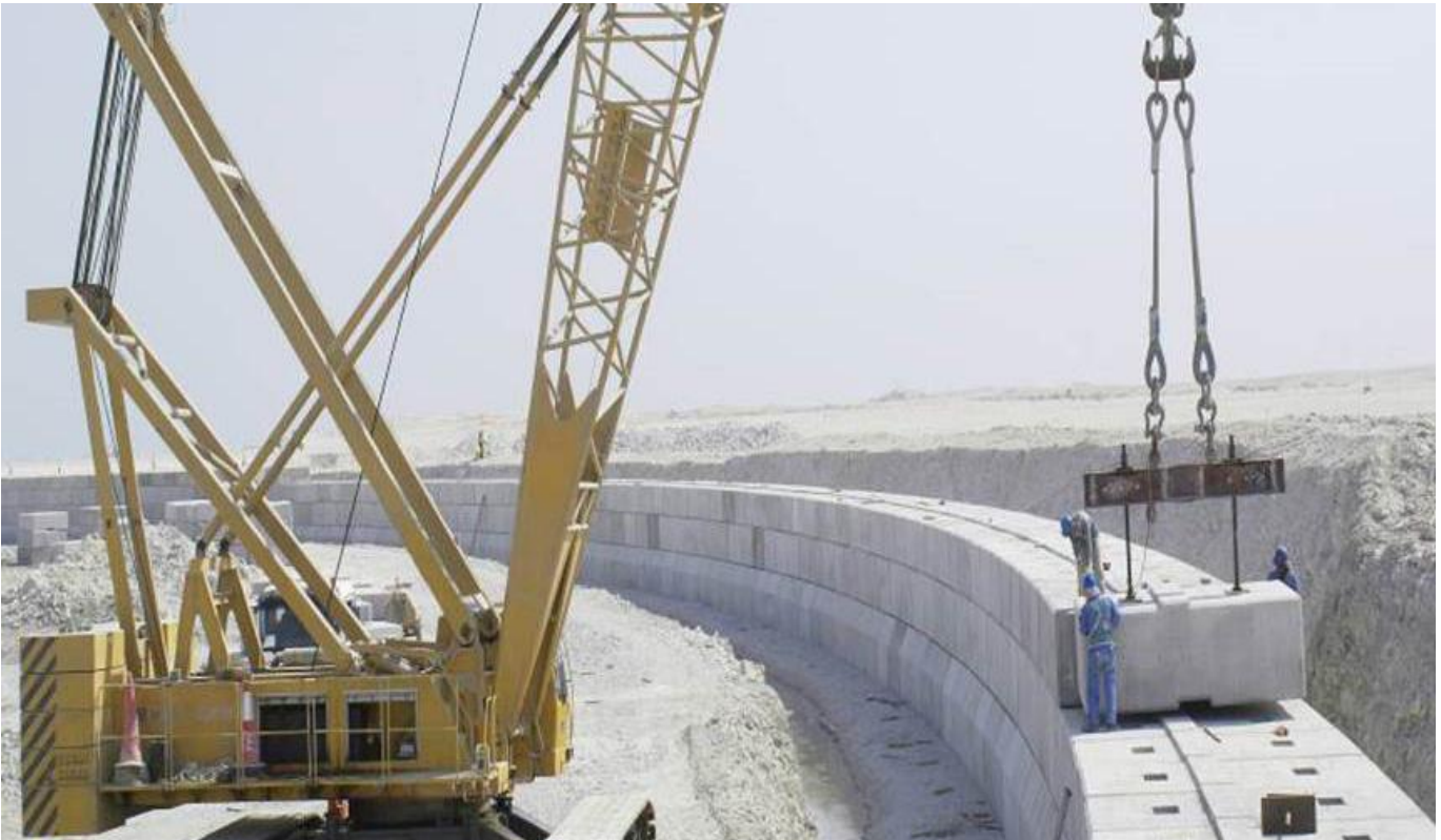
ERECTION OF PRECAST ELEMENTS – LUSAIL DEVELOPMENT PROJECT
